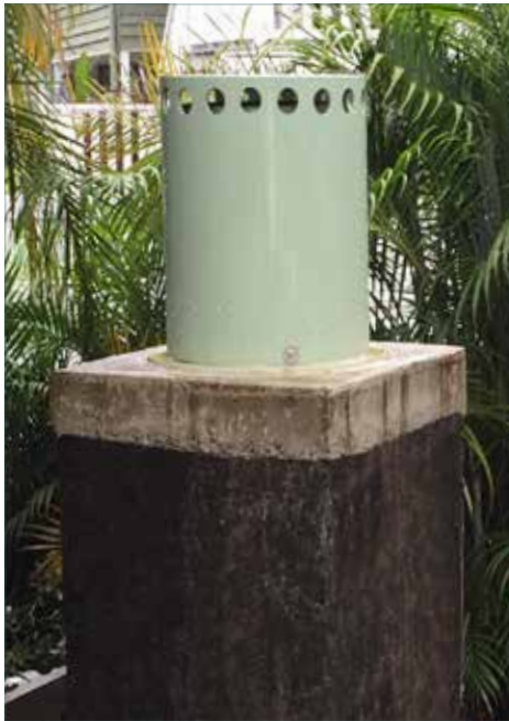
GM300 ON CUT-OFF CONCRETE VENT POLE
